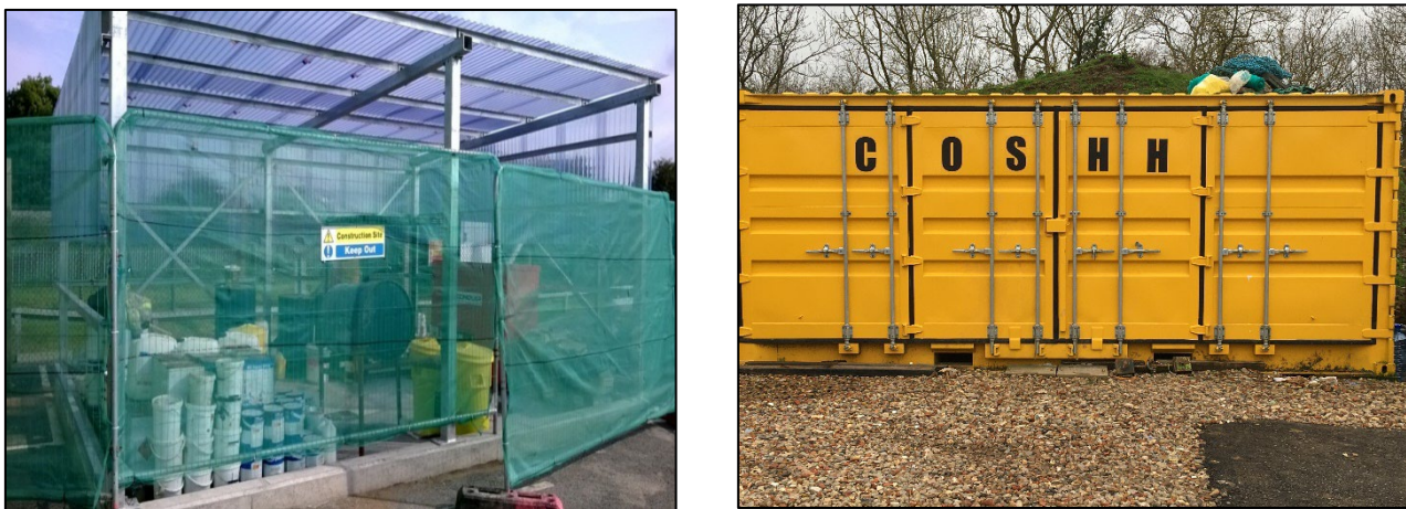
Figure 4 - Examples of bunded and covered COSHH areas and containers
